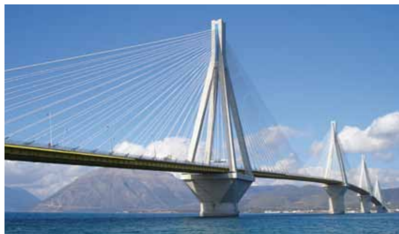
Harilaos Trikoupi Bridge, Greece
